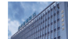
Anhui BAK New Power was registered successfully. In the June, it went into operation.
